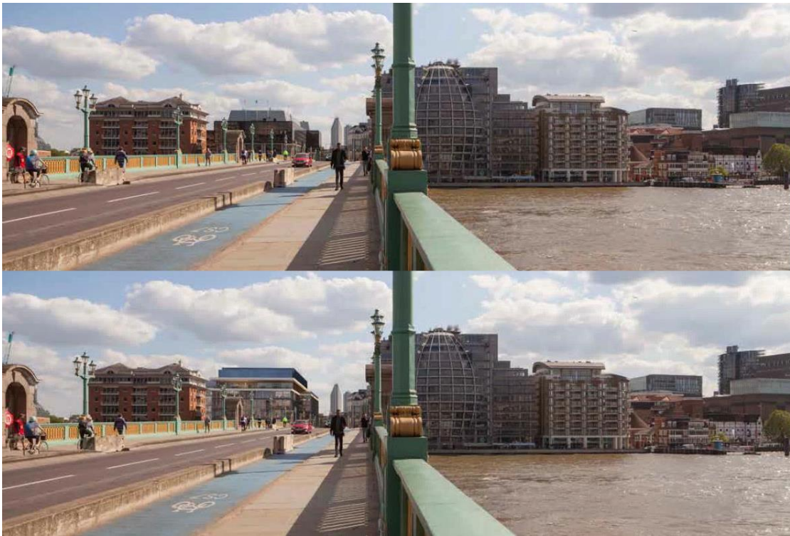
Figures 16 and 17 (above): The existing building (top) and proposal (bottom) as seen within the eastern portion of the LVMF River Prospect 12.A.
