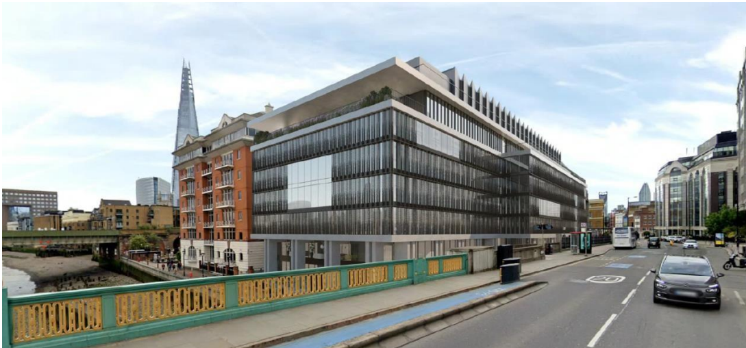
Figure 04 (above): View of the proposal, as seen looking southeastwards from Southwark Bridge.
